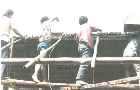
Lashing down the nabo 'roof'
