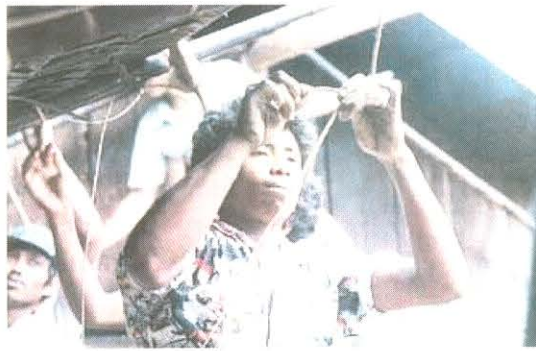
nabo 'roof' work
